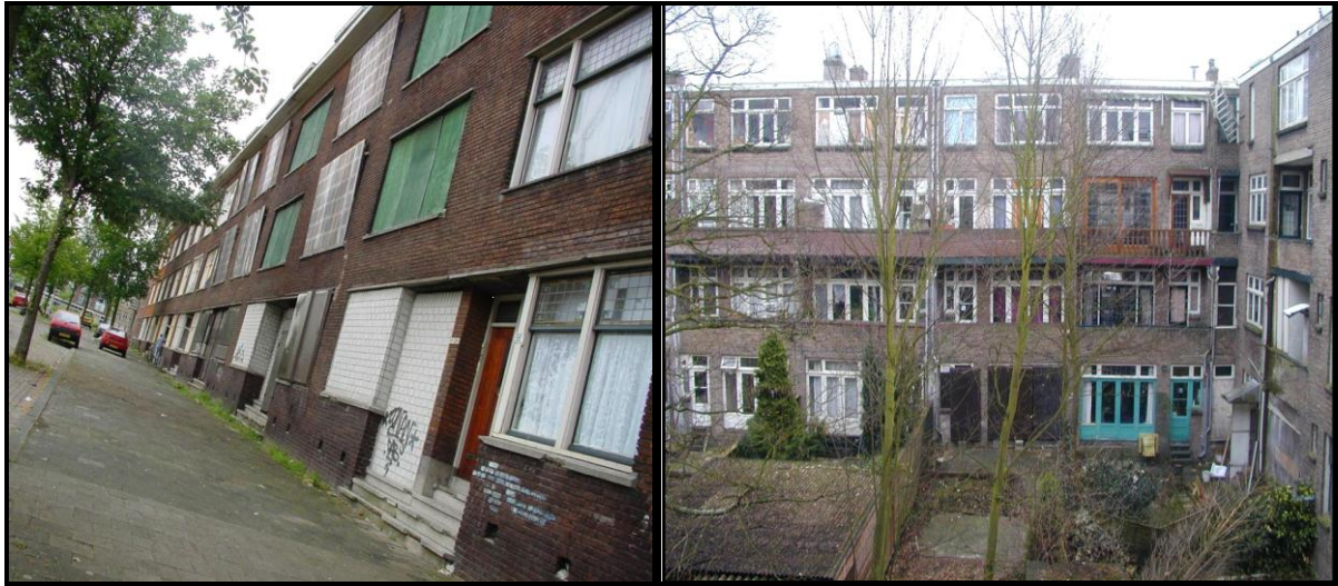
Figure 1: picture Wallisblok before renovation (2004)
